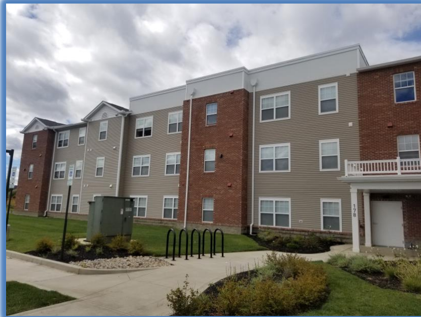
Wheatland Crossing is a combination of a garden apartments and townhomes.
