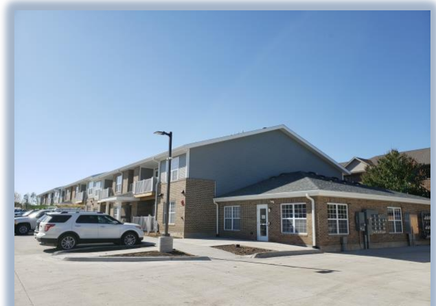
Anderson Greene, 69 Miller Ave, SW, Cedar Rapids, IA, is new 44-unit mixed income multifamily community soon opening in Cedar Rapids. A second phase offering 48 units is now under construction.
