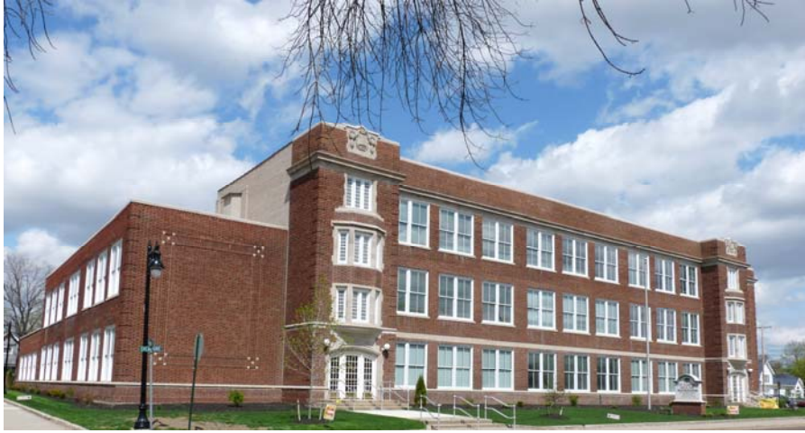
Sycamore House- A Woda Community
